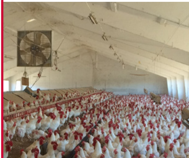
Figure 96 Circulation fans in an open-sided/naturally ventilated house.
