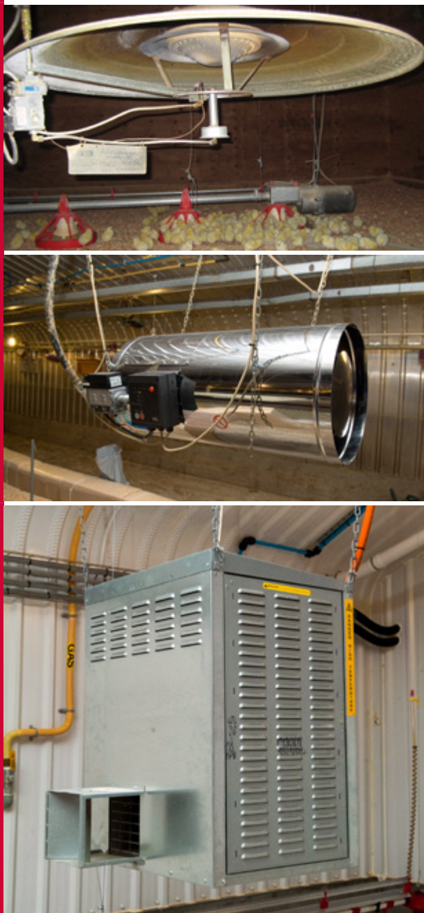
Figure 94 Examples of different house heating systems (from top to bottom, canopy brooder, whole-house heating and space heater).
