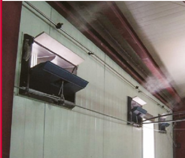
Figure 112 Example fogging system for a cross-ventilated house.
