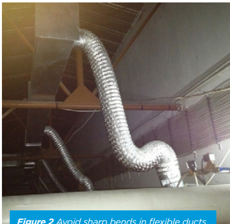
Figure 2 Avoid sharp bends in flexible ducts.
